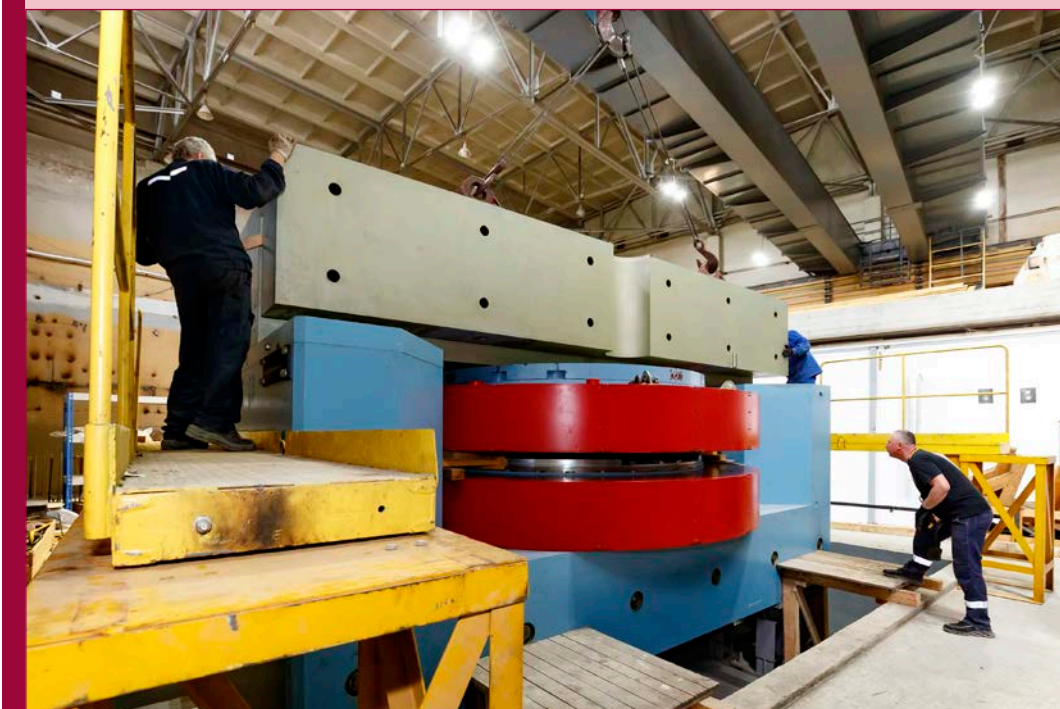
Installation of DC-140
